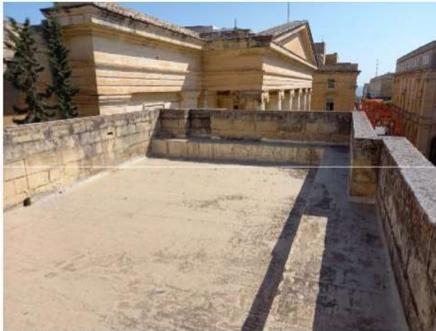
Pic 14 Rooftop adjacent to lawcourts
