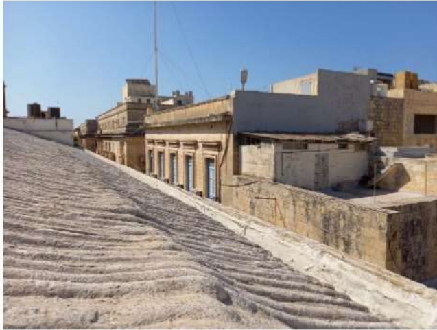
Pic 13 Roof top
