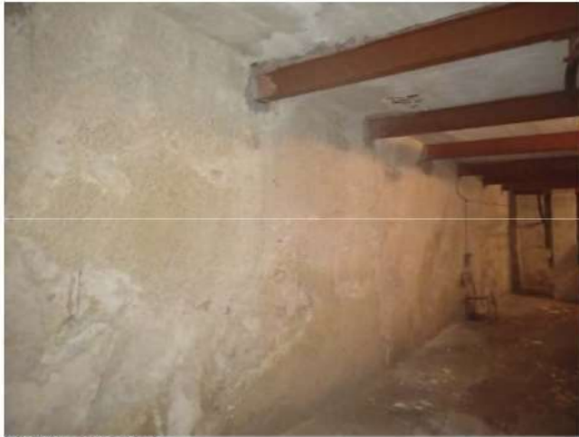
Pic 32 Underground area
