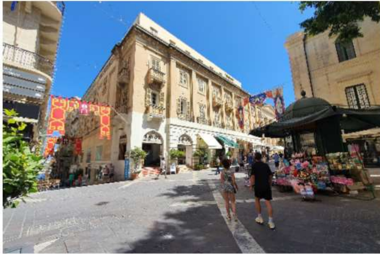
pic6 front facade from corner
