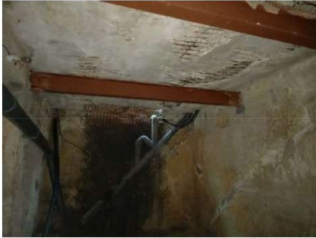
Pic 31 Underground area
