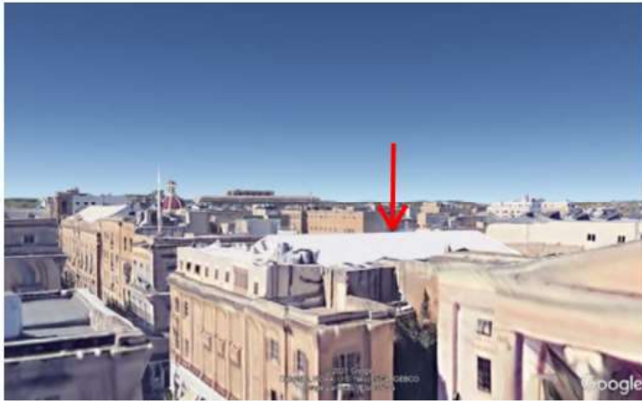
Pic 4. In red the apex of the steel roof structure
