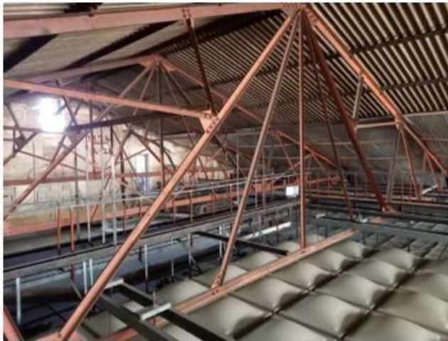
Pic 22 Internal view of roofing structure
