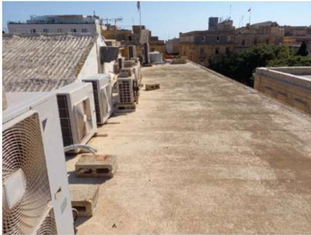
Pic 11 Rooftop & services
