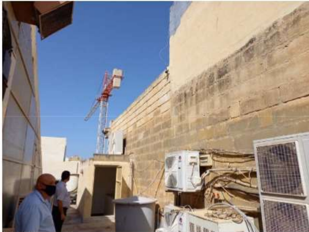
Pic 18 Internal shaft
