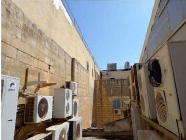
Pic 17 Internal shaft
