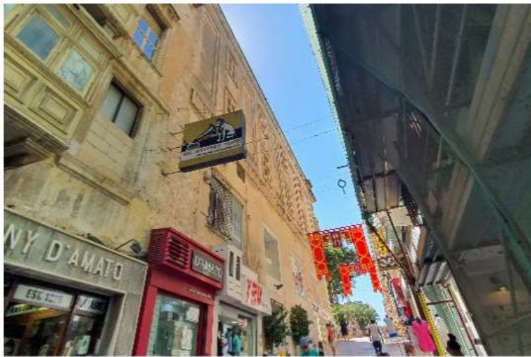
pic 7 side facade
