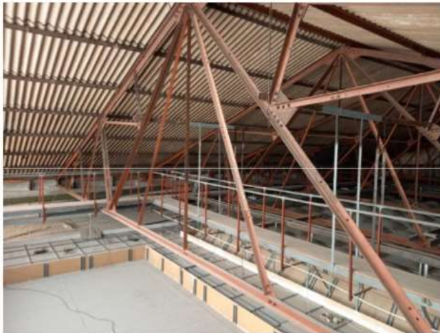
Pic 20 Internal view of roofing structure
