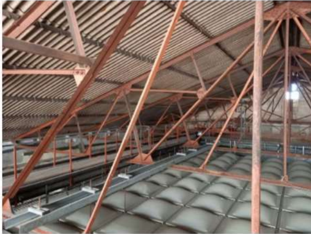
Pic 21 Internal view of roofing structure
